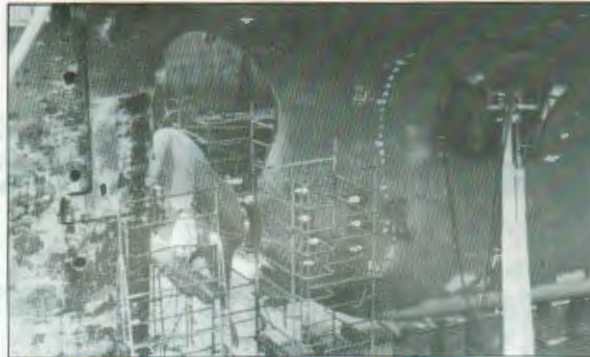
Preparation for taking out a tail shaft
