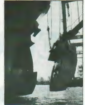
Removal of a 55-ton bulbous bow
