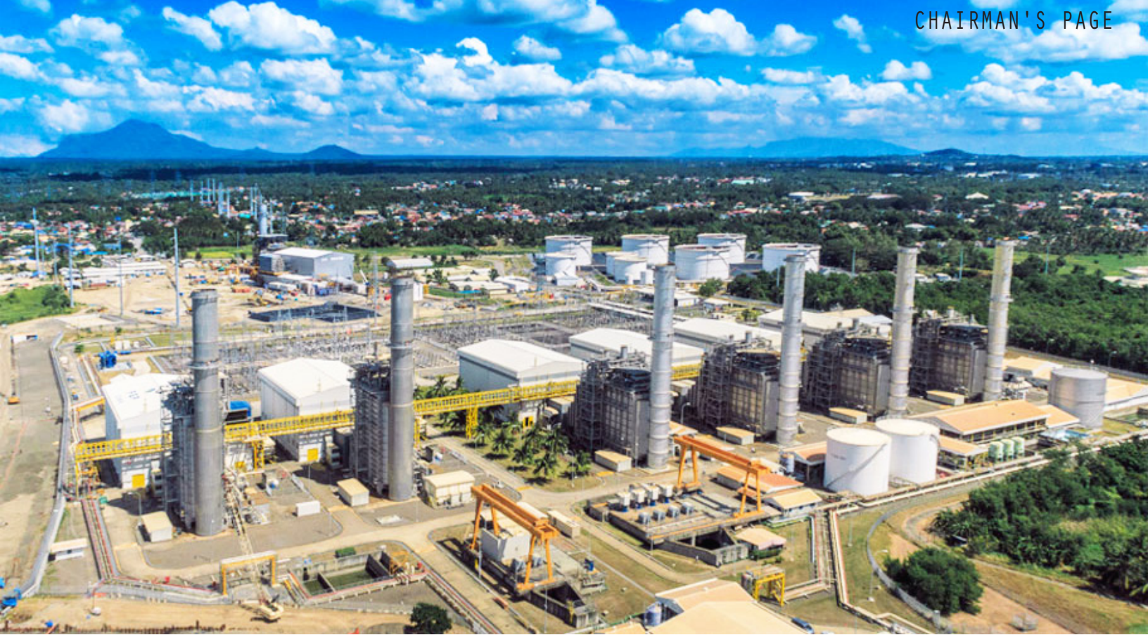
Photo: First Gen combined-cycle natural gas-fired power plant. Source: First Gen.
