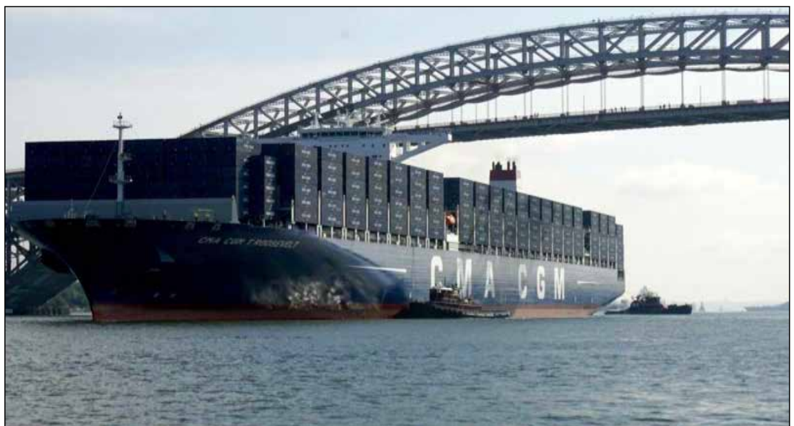
The raised Bayonne Bridge allows bigger ships to call at New York's terminals. Photo Credit: US Coast Guard/Sabrina Clarke
