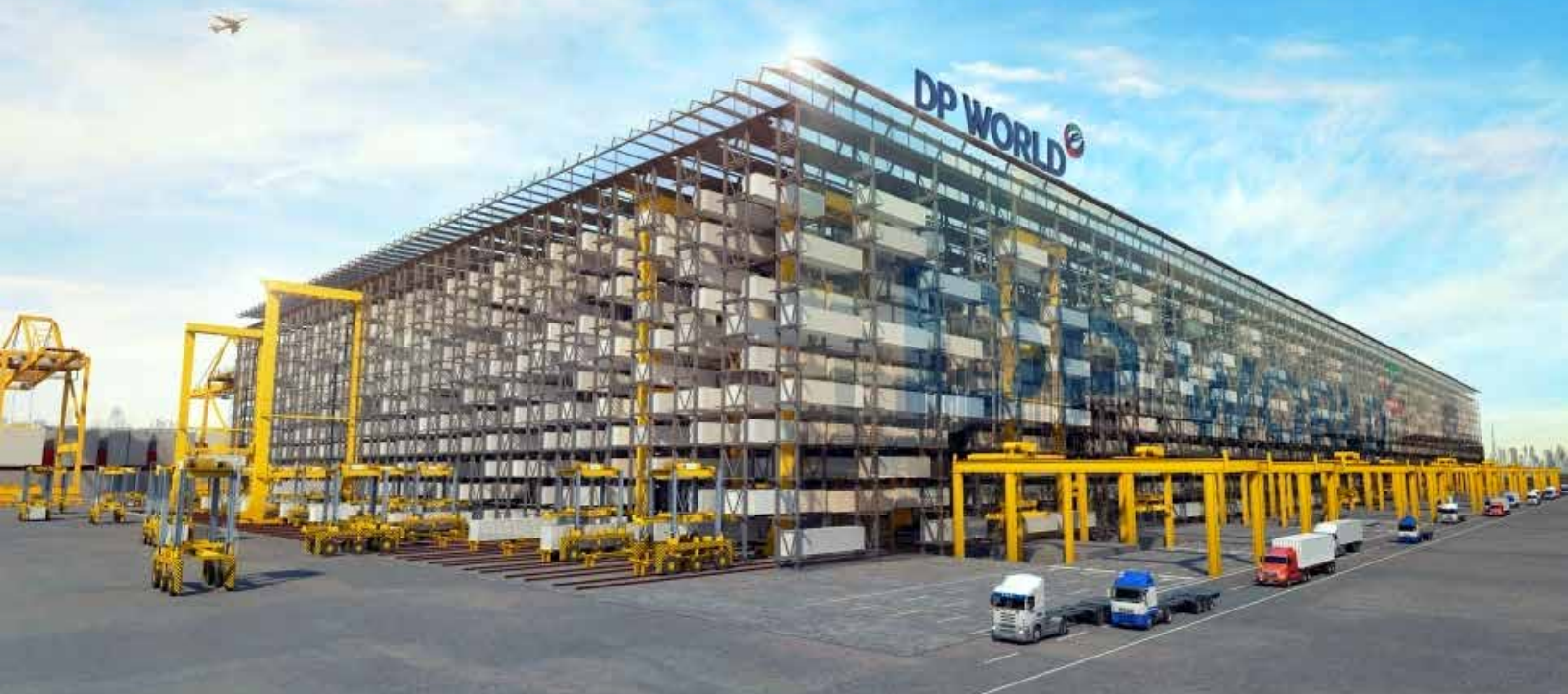
World's first high bay container storing system to be ready for 2020 World Expo in Dubai. Photo Credit: Saudi Gazette.
