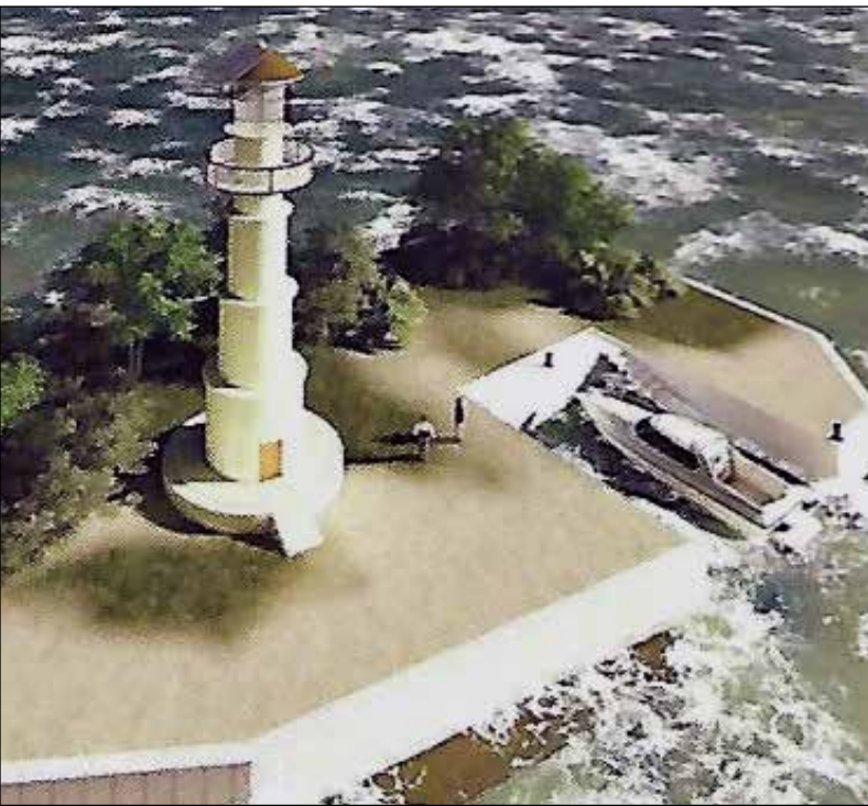
Design of the lighthouse with surrounding retaining walls to prevent erosion on the South Atoll of the Tubbataha Reefs Natural Park (TRNP) in Cagayancillo. Photo Credit: TRNP.
